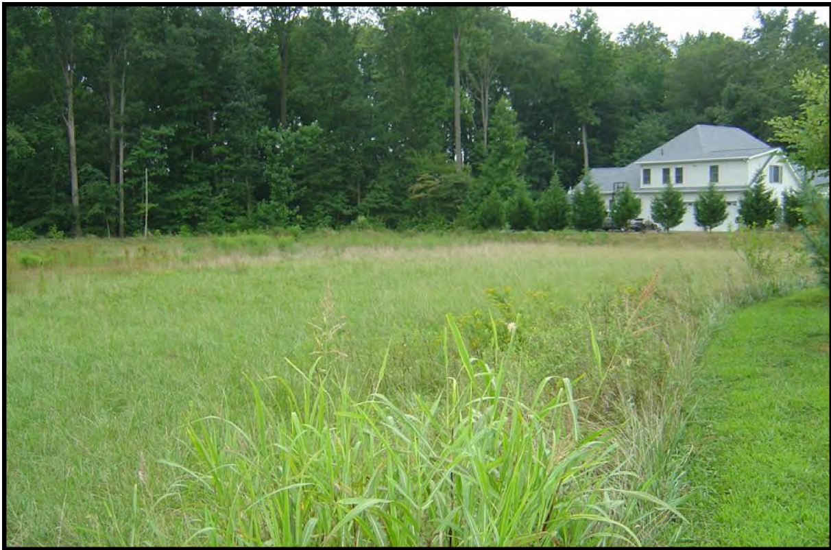
Figure 6.127: Extended Detention Wetland in a Residential Development. Dover, Delaware. Source: Kevin Magerr, PE, CPESC, CPSWQ.
