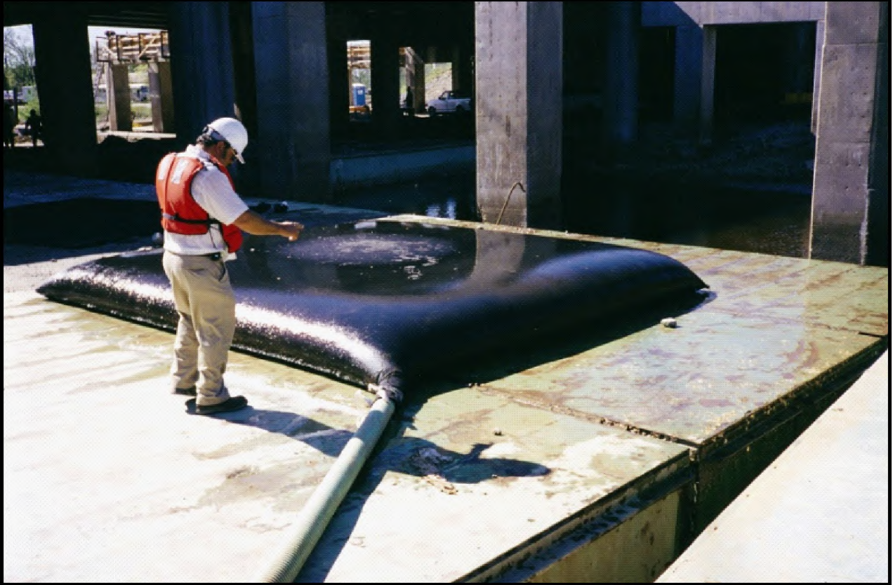
Figure 6.88 Use of a dewatering bag where storm water is pumped into a geotextile bag. The sediment stays in the bag while the storm water is allowed to flow out through the small voids in the material. Source: ACF Environmental Inc.
