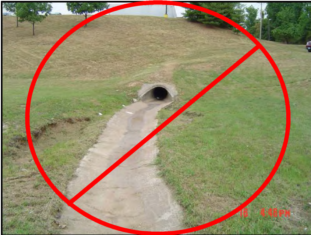
Figure 6.122 Detention basin with concrete conveyance channel. Source: Metropolitan St. Louis Sewer District
