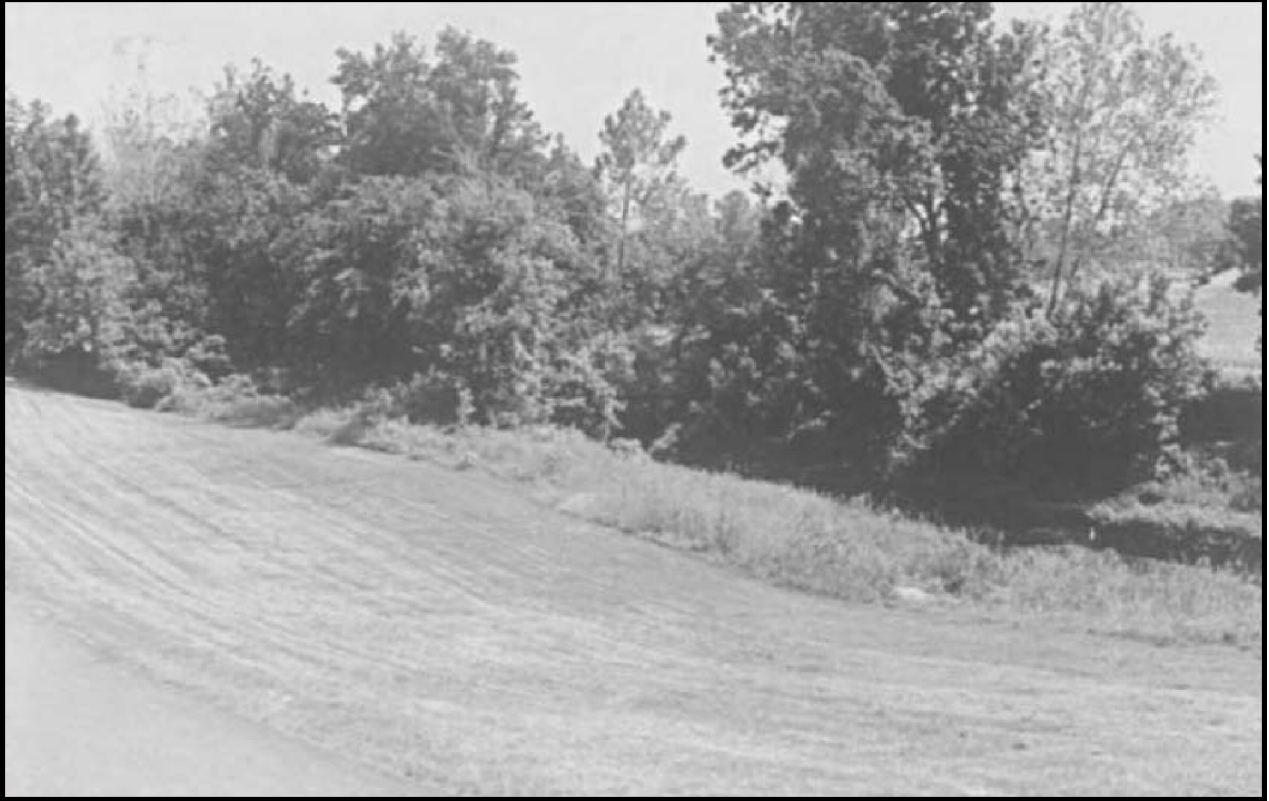
Figure 6.86 Vegetative buffer strips slow surface runoff, reduce sedimentation and help capture pollutants. Depending on the choice of plant materials, they can be low maintenance areas (mow once or twice a year) or provide habitat for wildlife.
